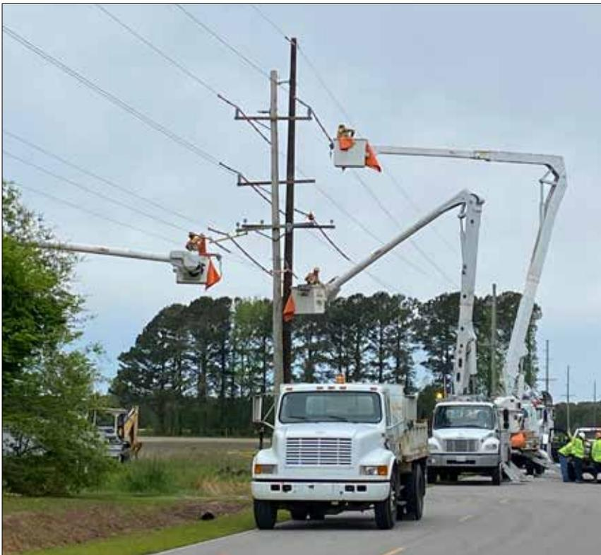
MasTec construction crews prepare to place protective rubber sleeves on the energized line so they can begin work on new iron pole installation.
