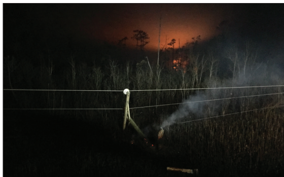
Tideland pole succumbed to the Whipping Creek Fire in April 2016. Photo by Justin Gibbs, Hyde County Emergency Services
