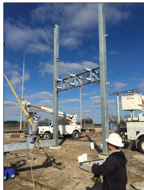
Engelhard substation construction
