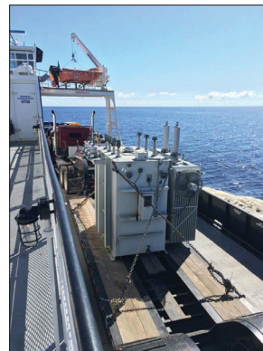
Emergency transformer transport
