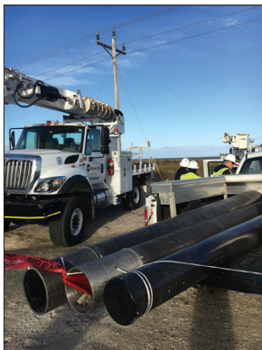
Intelli-pole installation at Ocracoke
