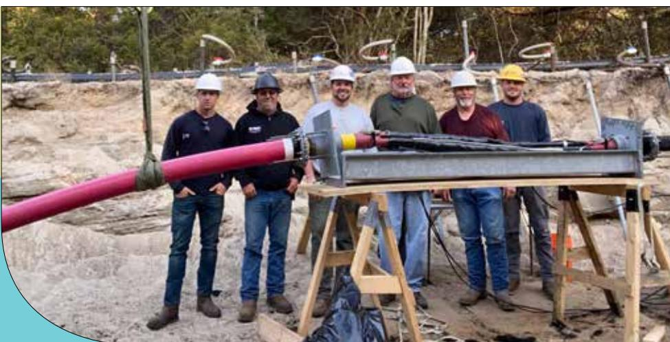
On March 19, crews completed splicing and successfully energized the new submarine cable on the south end of Hatteras Island. This \$3.5 million project ensures continuity of service to Ocracoke in the face of continued erosion and encroaching seas. The existing overhead line will be removed, allowing the area to return to its natural vegetative state.
