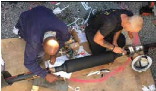
Splicing experts repair the first line. As excavation continued for the third cable the site filled with water.
