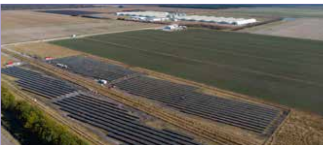
North Carolina Electric Membership Corporation Microgrid at Rose Acre Farms
