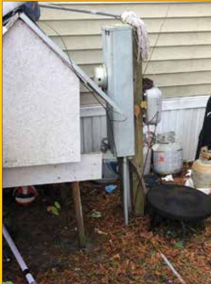
Needs to declutter area around meter base
