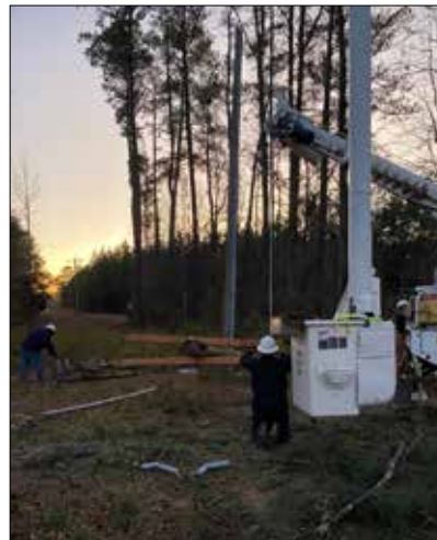
Bonnerton circuit repairs near Ephesus Church Road (Wayne Brackin photo)
