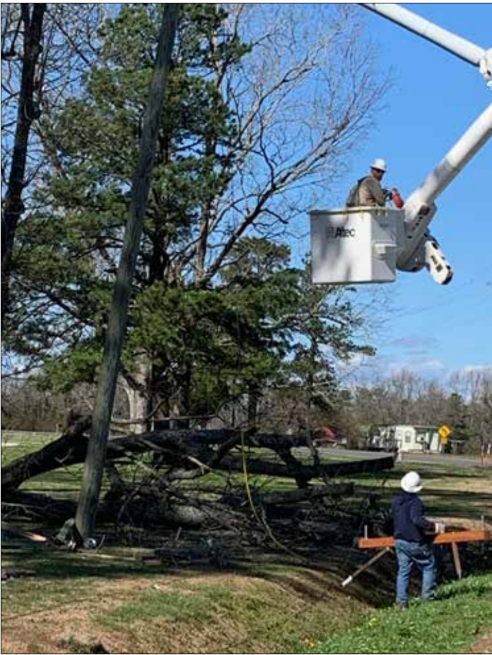
Linemen Jacob Hardison and Robert Shively replace broken crossarms on Free Union Church Road. Paul Spruill photo
