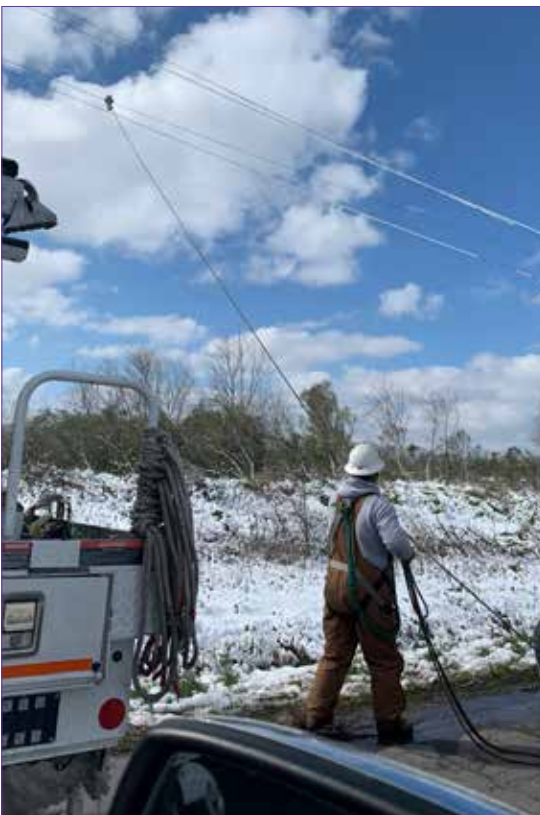
Lineman Josh Dunbar uses a wire pulley to de-ice a line. Paul Spruill photo
