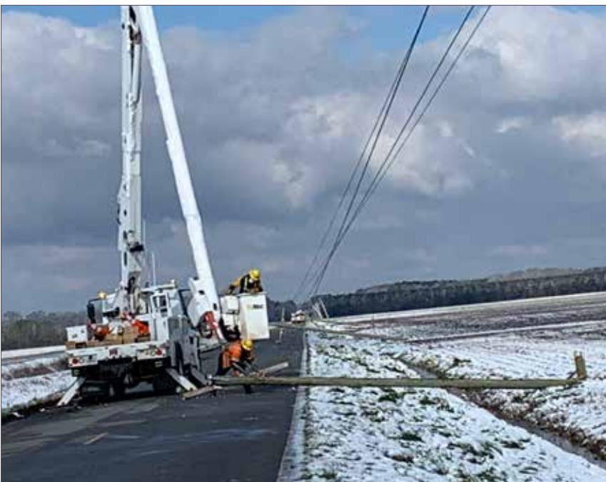
Galloping lines brought down ten poles on this stretch of Old Hwy 97. Paul Spruill photo
