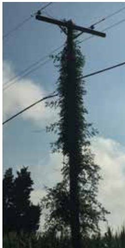
Warmer temperatures and higher humidity levels have extended growing seasons leading to explosive vine growth
