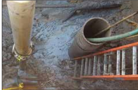
Splicing experts repair the first line. As excavation continued for the third cable the site filled with water.
