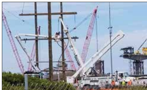
Ultimately, the overhead solution crossed the finish line first with transmission restored on August 3
