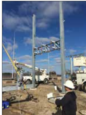
Engelhard substation construction
