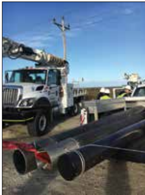
Intelli-pole installation at Ocracoke
