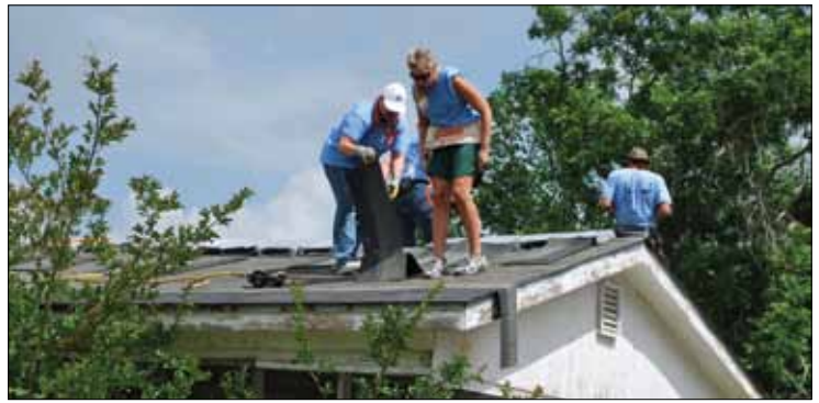
Volunteers re-shingle Rachel Alston’s roof
