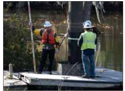
RIVER CITY CONSTRUCTION CREWS INSTALL CAISSONS AND DUCTILE POLES ALONG BROAD CREEK ROAD IN WASHINGTON. JIM CHRISMAN PHOTOS
