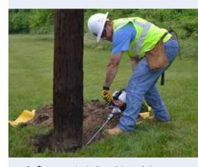
An Osmose contractor bores into a pole to inspect for internal signs of decay.
