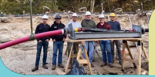
On March 19, crews completed splicing and successfully energized the new submarine cable on the south end of Hatteras Island. This \$3.5 million project ensures continuity of service to Ocracoke in the face of continued erosion and encroaching seas. The existing overhead line will be removed, allowing the area to return to its natural vegetative state.
