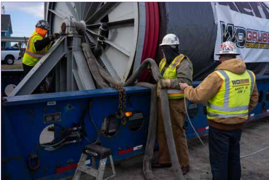
In this series of photos, the cable is readied for off-loading from the transport vehicle. Cranes transferred it to a modified
