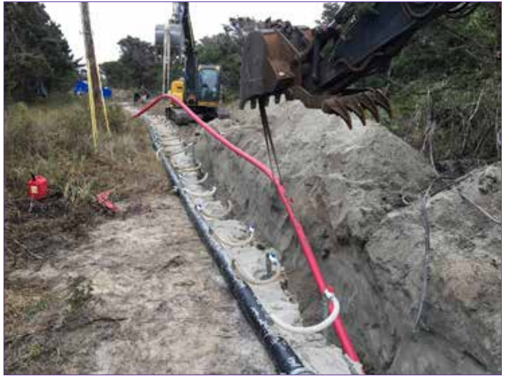
Trenching and dewatering work underway. Ben Beagle photo
