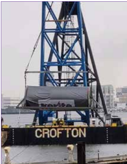
The cable arrives in Virginia. Kerite photo
