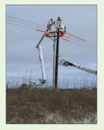
assembly, it can be transported in the back of a pickup truck and hand carried into tight locations. It will not rot, corrode or decay, and is 100% recyclable. Best of all it is rated to withstand winds in excess of 180 miles per hour. Tideland's engineering team chose to install the pole in an area that is most frequently subjected to straight line winds and ocean overwash.
