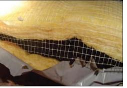
Damaged ductwork, like this found in a Tideland member's attic, is frequently found to be the cause of high bills. *Larry Johnson/TEMC photo*
